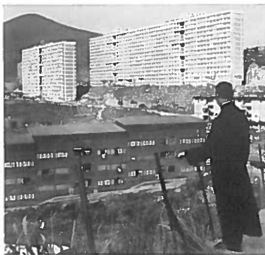
Caracas (Venezuela): Holzhäuser und Wohnblocks unserer Pfarrei in Caracas - Frame houses and residential blocks of our parish.
